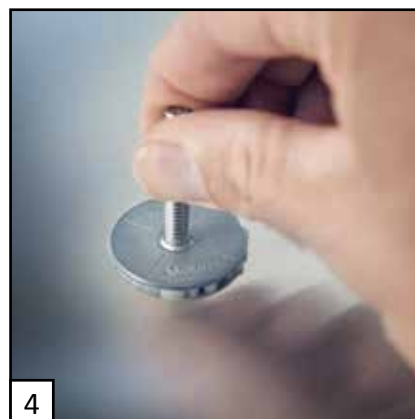
4 Firmly push the part onto the substrate until the adhesive squeezes out from under the base. Depending on the adhesive selected the fastener is ready for use in 15 - 45 minutes.
